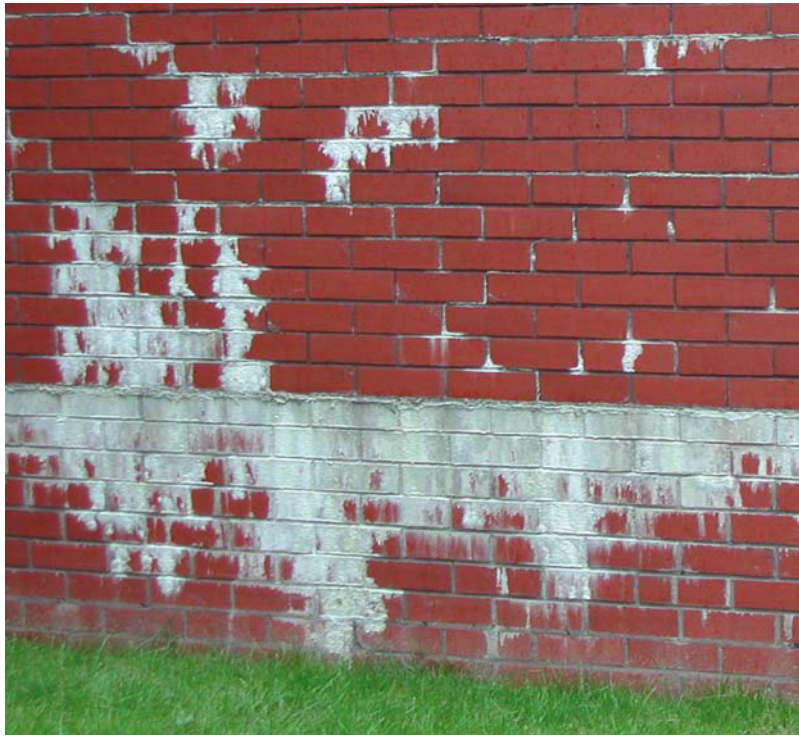
Fig. 1.14 Lime leaching on brickwork
