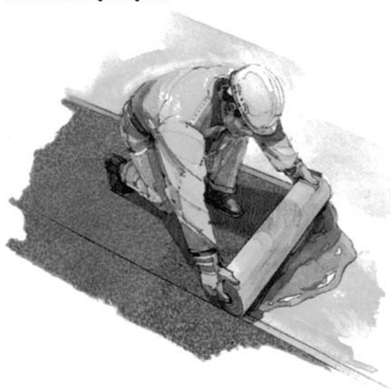
Torching-on high-performance roofing sheet
