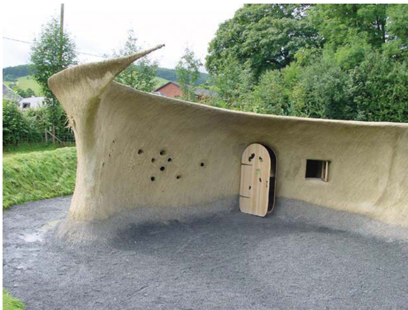
Fig. 17.4 Mud and straw construction—The House for Stories, Bledfa Centre for the Arts, Powys, Wales. Architect: Tono Mirai. Photograph: Courtesy of Richard Weston
