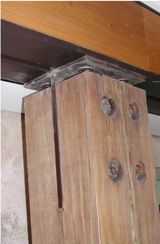
Fig. 4.28 Laminated timber beam metal joint detail—Wells Cathedral Restaurant. Photograph: Arthur Lyons
