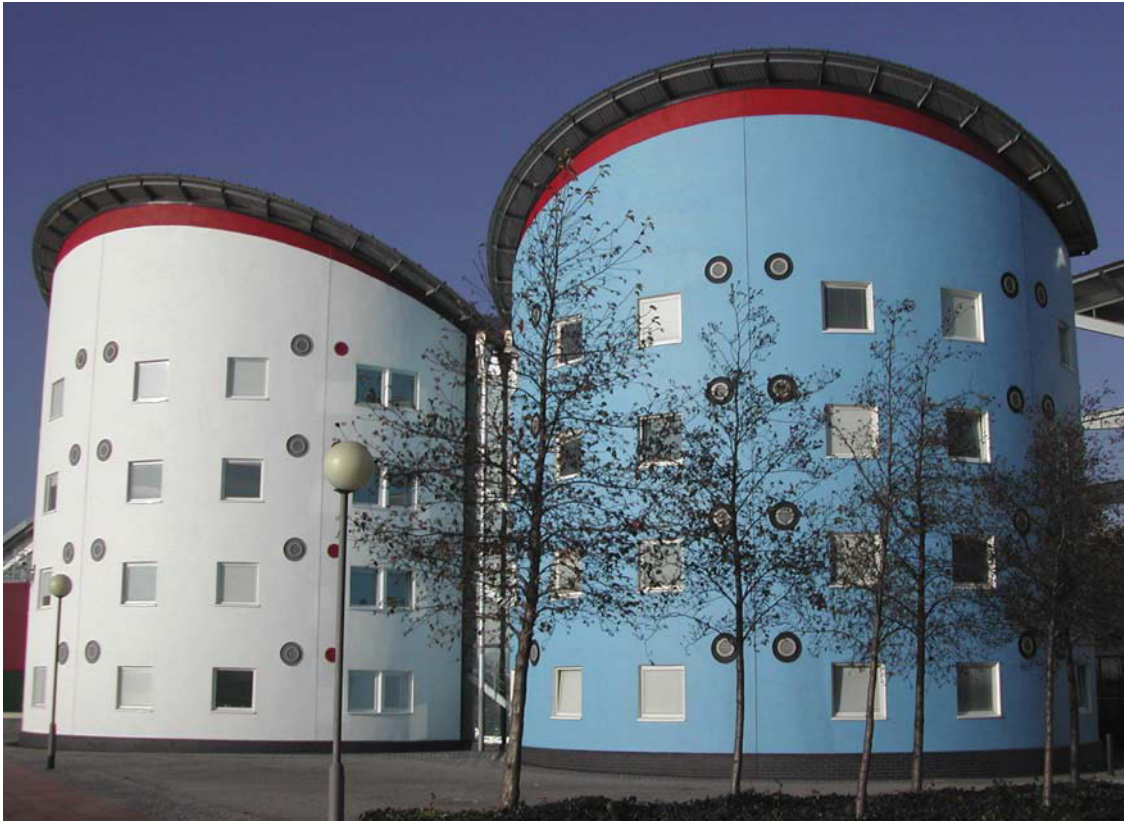
Fig. 3.26 Rendered blockwork — University of East London, Docklands Campus. Architects: Edward Cullinan Architects. Photograph: Arthur Lyons
