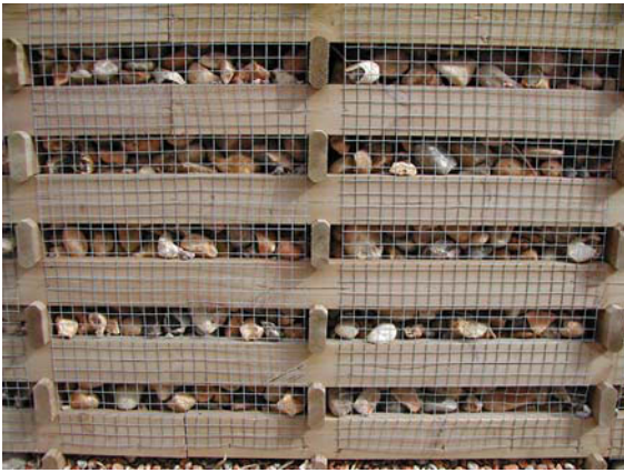
Fig. 9.16 Timber mesh and stone earth-retaining system
