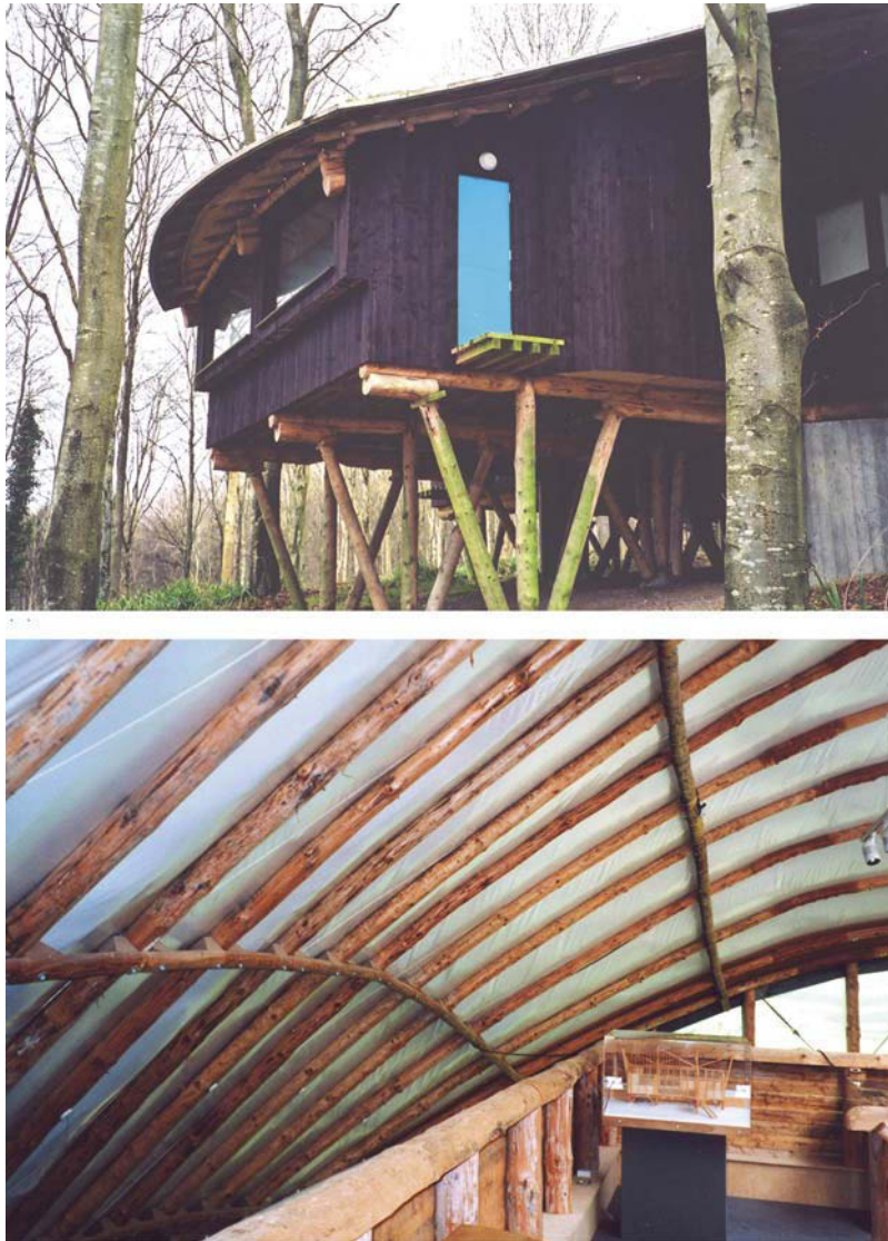
Fig. 4.19 Timber pole construction—Hooke Park, Dorset—lodge (Edward Cullinan Architects and Buro Happold), and workshop interior (Frei Otto, Ahrends Burton and Koralek and Buro Happold). Photographs: Courtesy of Allan Glennie
