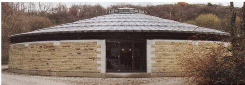
Fig. 9.14 Load-bearing stone masonry—David Mellor Cutlery Factory, Hathersage, Derbyshire. Architects: Hopkins Architects. Photographs: Arthur Lyons
