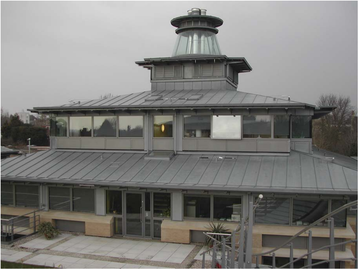
Fig. 5.30 Zinc alloy roofing—Centre for Mathematical Sciences, University of Cambridge. Architects: Edward Cullinan Architects. Photograph: Arthur Lyons
