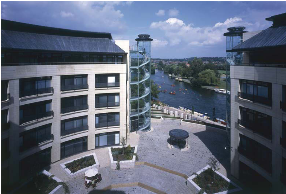
Fig. 9.21 Reconstructed stone cladding—Thames Water, Reading. Photograph: Courtesy of Trent Concrete Ltd
