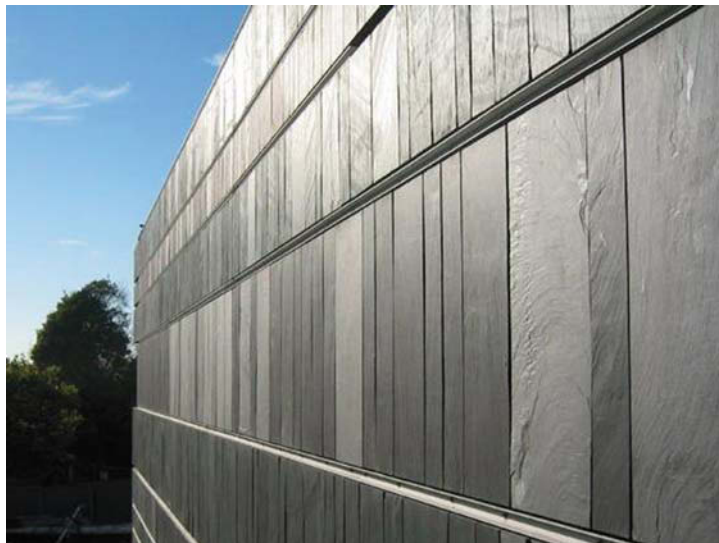
Fig. 3.20 Slate surfaced precast concrete cladding—Swansea Museum. Photograph: Courtesy of Trent Concrete Ltd.
