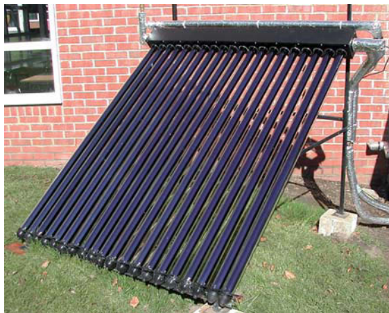
Fig. 16.4 Evacuated-tube solar collectors
