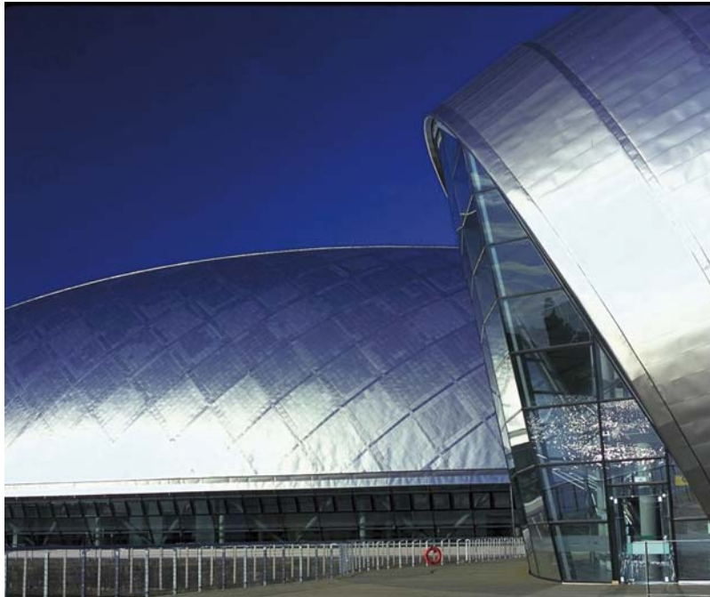
Fig. 5.32 Titanium cladding—the Glasgow Science Centre. Architects: BDP, Building Design Partnership. Photograph: Courtesy of Don Clements
