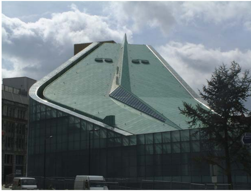
Fig. 5.23 Copper roof construction—Urbis Centre, Manchester. Architects: Ian Simpson Architects. Photograph: Courtesy of Chris Hodson
