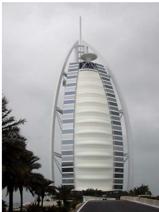
Fig. 10.14 Teflon-coated glass fibre membrane — Burj Al Arab Hotel, Dubai. Architects: WS Atkins. Photograph: Athur Lyons
