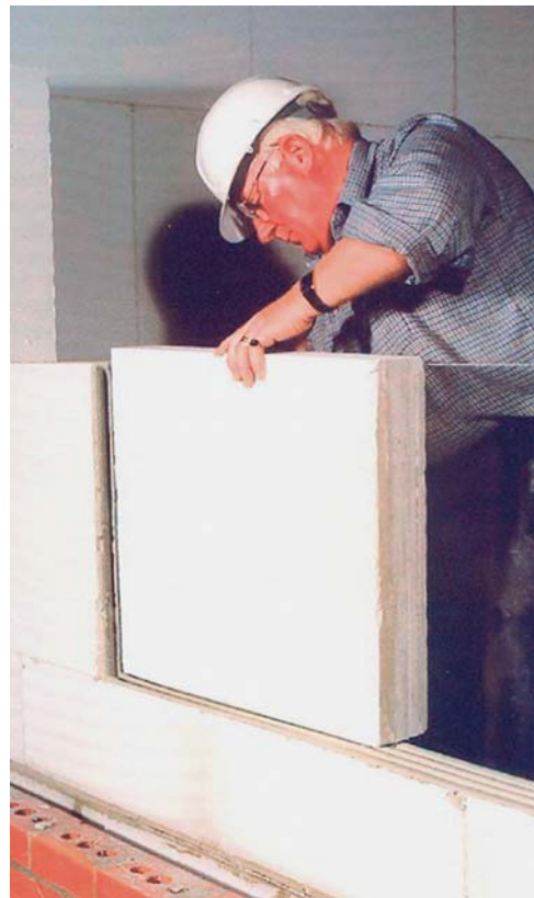
Fig. 2.3 Thin-joint masonry using large format blocks. Photograph reproduced from GBG 58 by permission of BRE and courtesy of Aircrete Products Association
