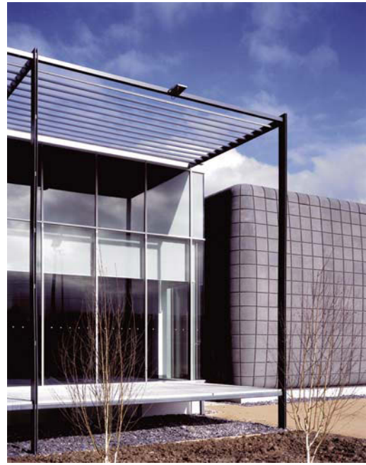
Fig. 3.21 Reconstructed stone cladding—Experian Data Centre, Nottingham. Photograph: Courtesy of Trent Concrete Ltd.
