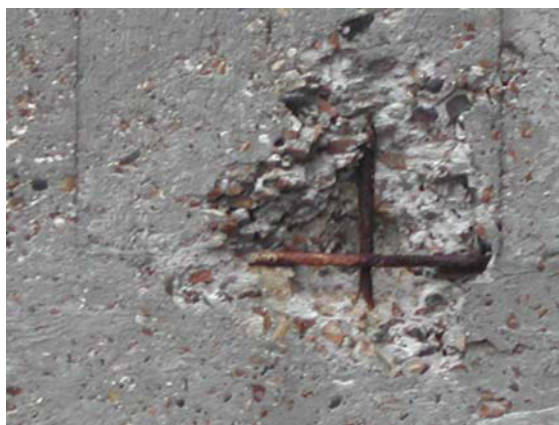
Fig. 3.16 Corrosion of steel reinforcement
