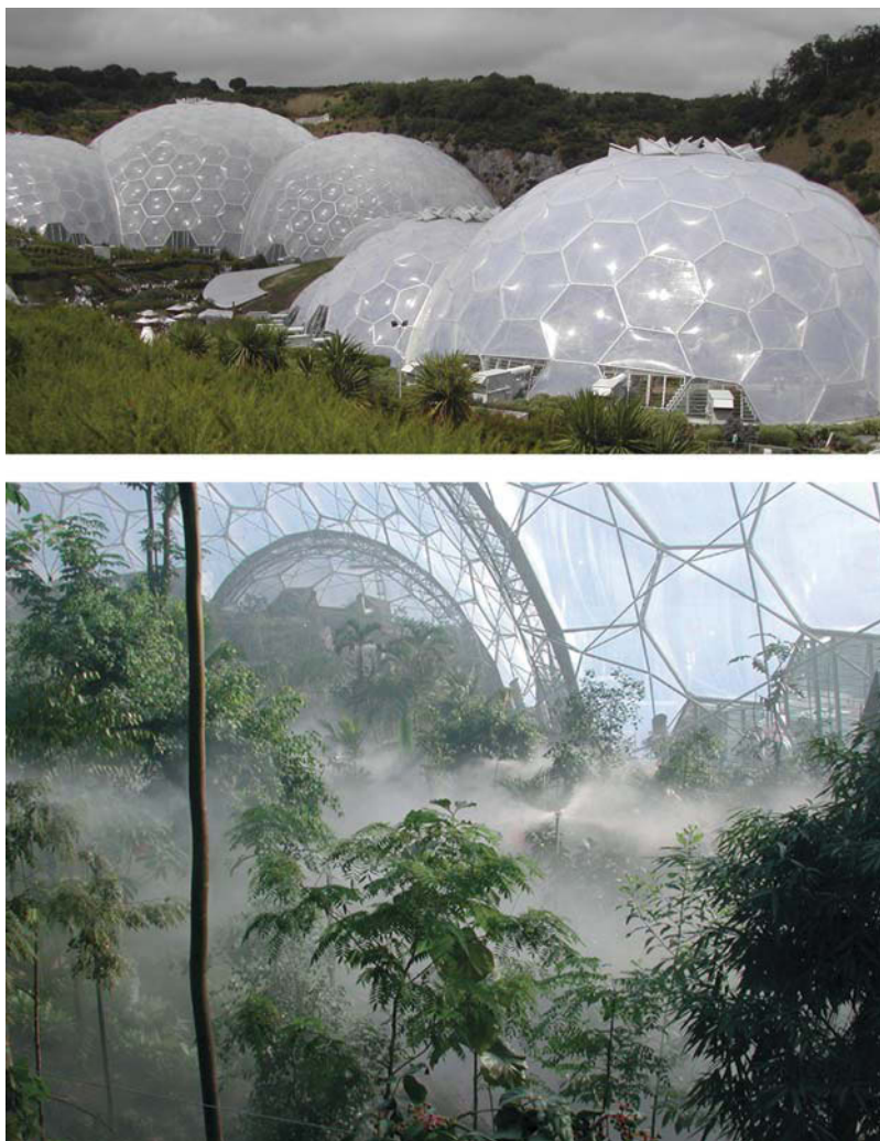
Fig. 10.15 ETFE—Eden Project, Cornwall. Architects: Grimshaw Architects. Photographs: Arthur Lyons and courtesy of Perry Hooper (interior)
