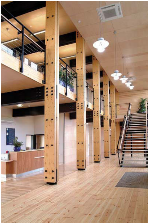
Fig. 4.30 Laminated veneer lumber (LVL) construction — Finnforest Office, Boston, Lincolnshire. Architects: Arosuo and Vapaavuori Oy. Photograph: Courtesy of Finnforest
