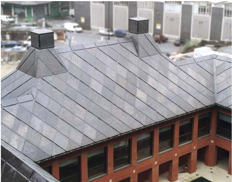
Fig. 5.29 Lead tile roofing—Haberdashers’ Hall, London. Architects: Hopkins Architects. Photograph: Courtesy of Lead Contractors Association
