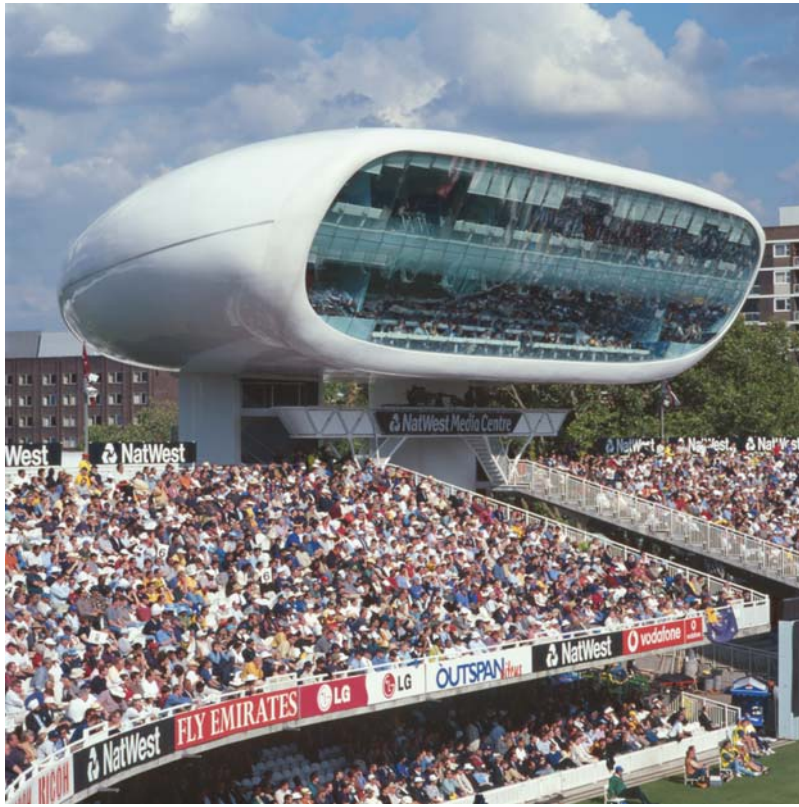
Fig. 5.21 Aluminium semi-monocoque construction—Lord's Media Centre, London. Architects: Future Systems. Photograph: Courtesy of Richard Davies
