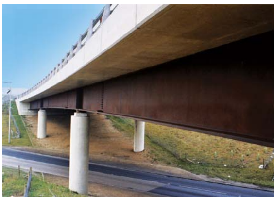
Fig. 5.16 Corten weathering steel—Chieveley interchange. Photograph: Courtesy of Corus
