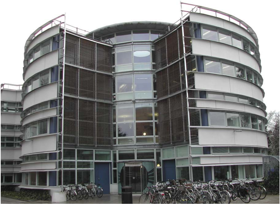
Fig. 5.19 Aluminium shading devices — Faculty of Divinity, University of Cambridge. Architects: Edward Cullinan Architects. Photograph: Arthur Lyons
