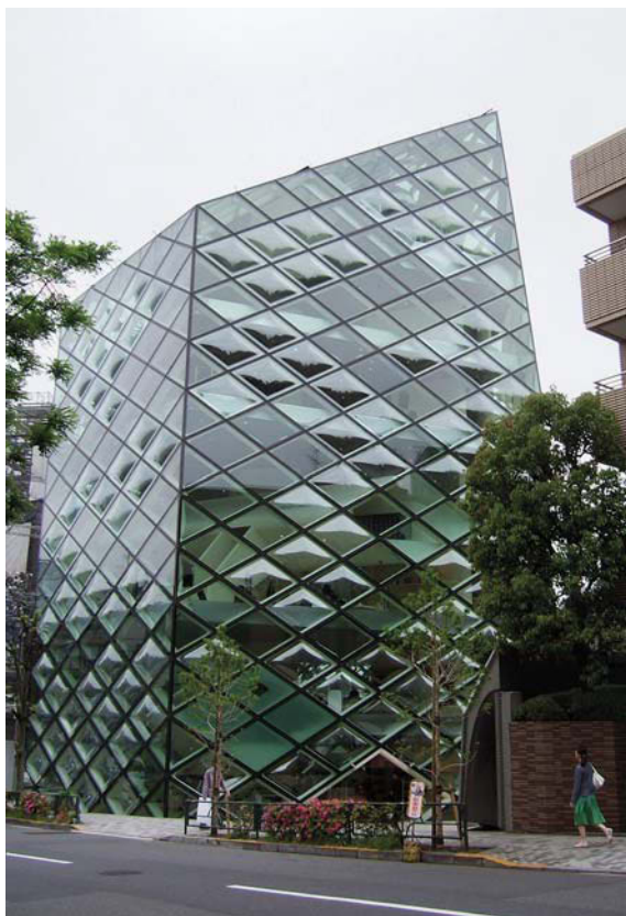
Fig. 7.14 Curved rhomboidal glass panes—Prada Store, Tokyo. Architects: Herzog & de Meuron. Photograph: Courtesy of Sam Glynn
